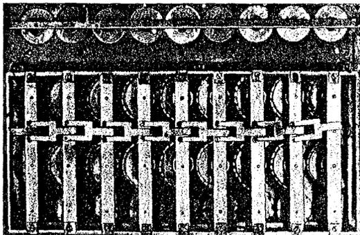
Fig. 2 The mechanism of Jakobson's machine
